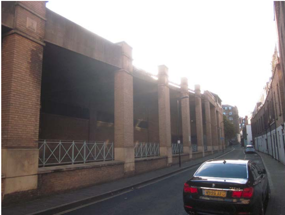
Front (west) elevation at corner of Queensway and Porchester Gardens (top) and rear (east) elevation in Redan Place (bottom).
