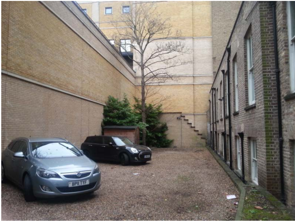
View from Redan Place (top) and eastward view within existing yard area (bottom).
